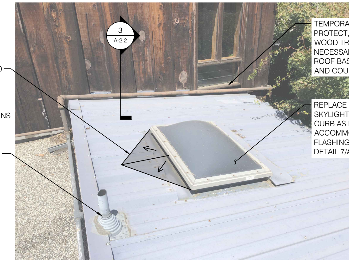
4 Main House (Primary Bathroom) Roof - Existing Conditions Not to Scale
