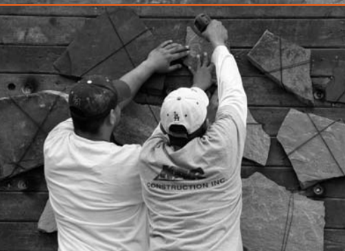
Building progress on schedule
