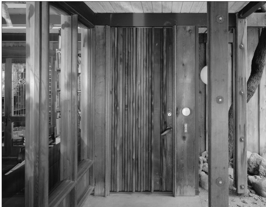
Image 14: Main House, east elevation, view west (HABS, 2003)
