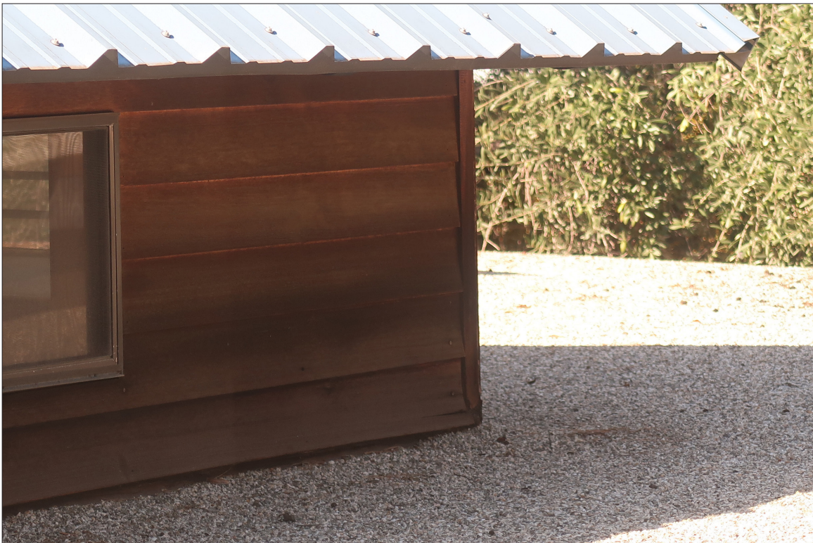
Image 22: Detail of horizontal wood siding (Chattel, 2022)
