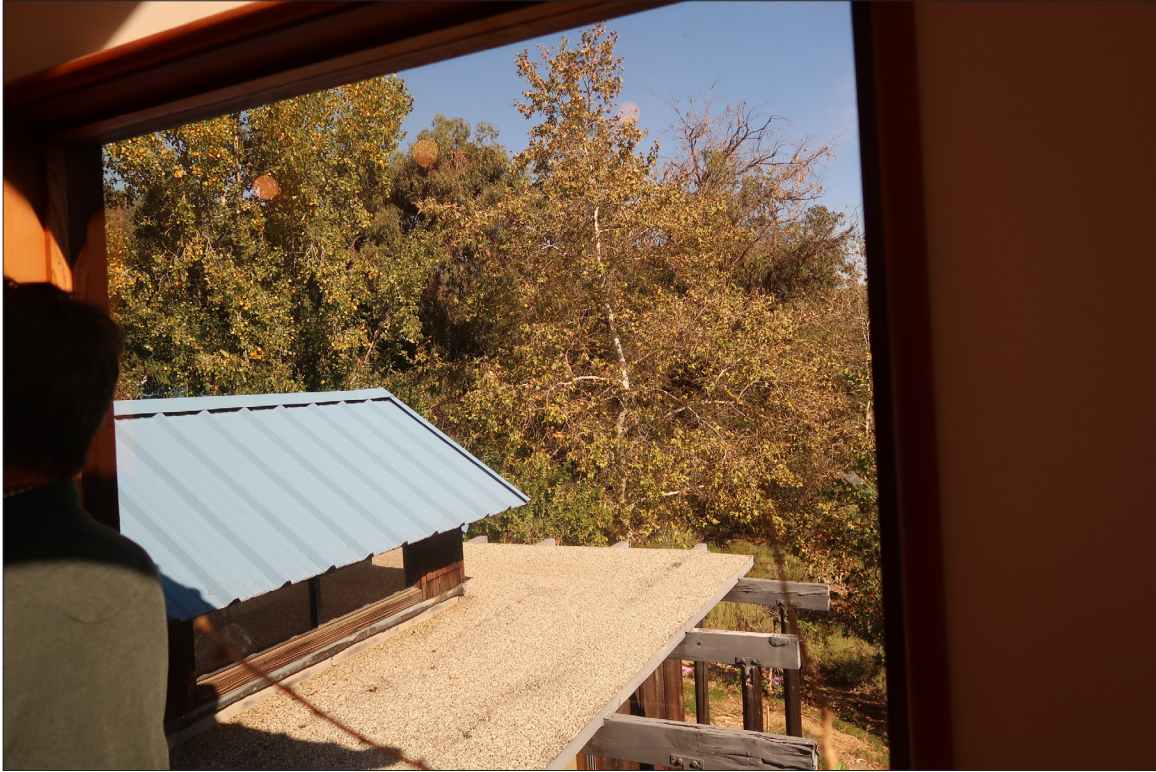
Image 19: Main House, built-up asphalt roof with gravel surfacing, view east (Chattel, 2022)
