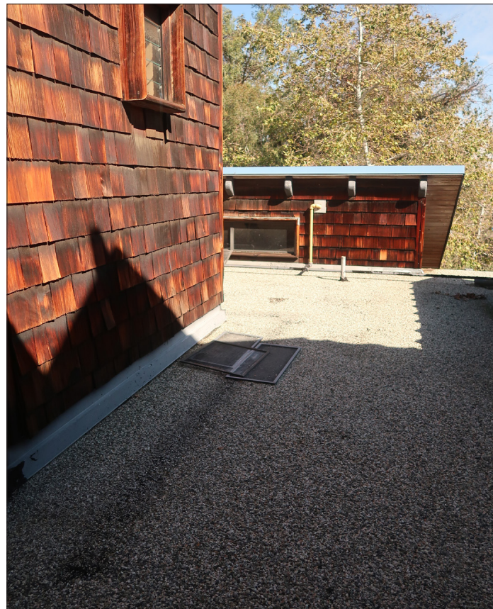
Image 20: Main House, built-up asphalt roof with gravel surfacing, view east. Note wood shake siding. (Chattel, 2022)
