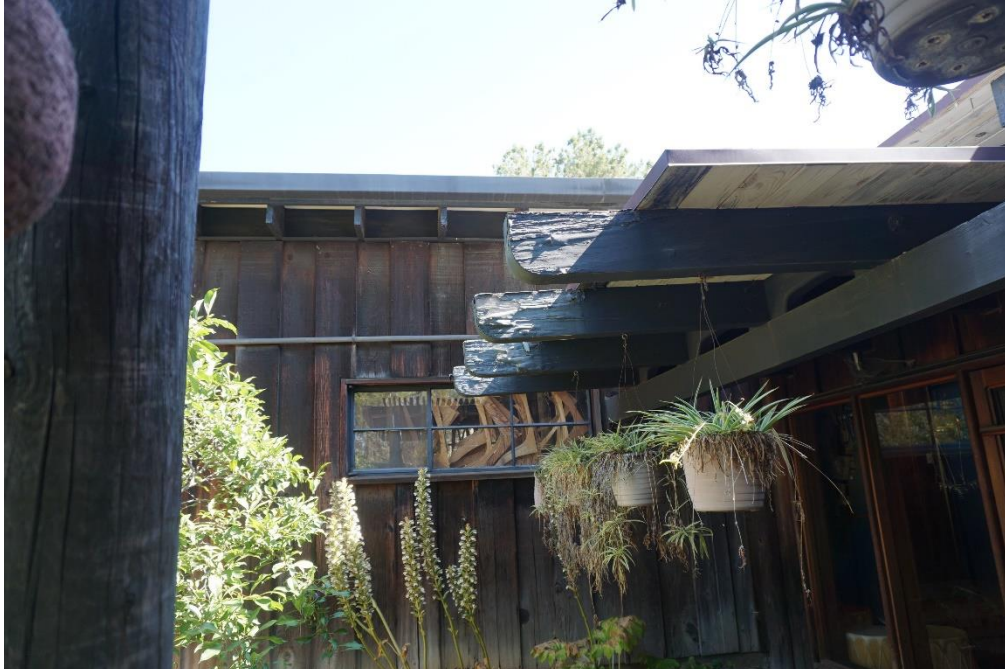
Figure 28. Example of typical low visibility of metal roofing from grade.
