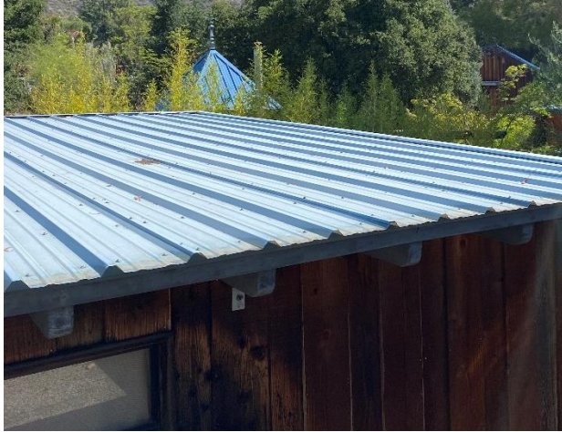
Figure 12. Existing metal panel roof profile
