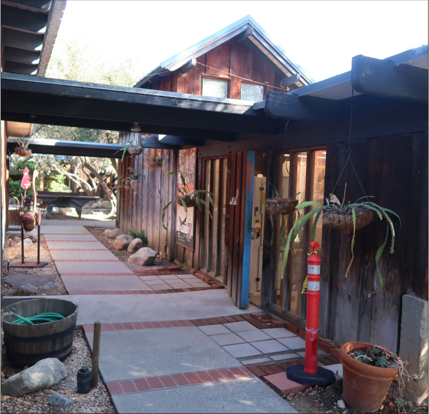
Image 5: Workshop 1 (right) and Workshop 2 (left), view east (Chattel, 2022)
