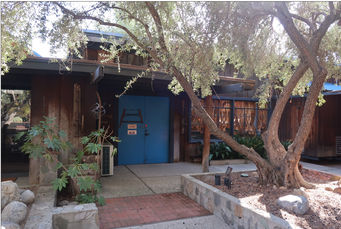
Image 3: Workshop 2, east elevation, view west (Chattel, 2022)
