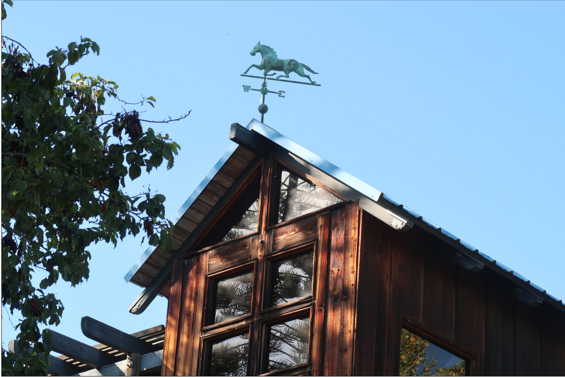
Image 9: Main House, south elevation, view northwest (Chattel, 2022)
