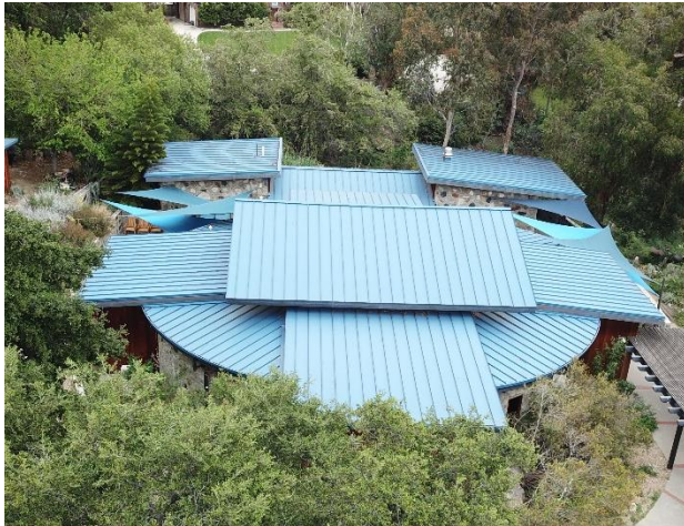
Figure 14. Existing standing seam metal roofs at the Maloof complex
