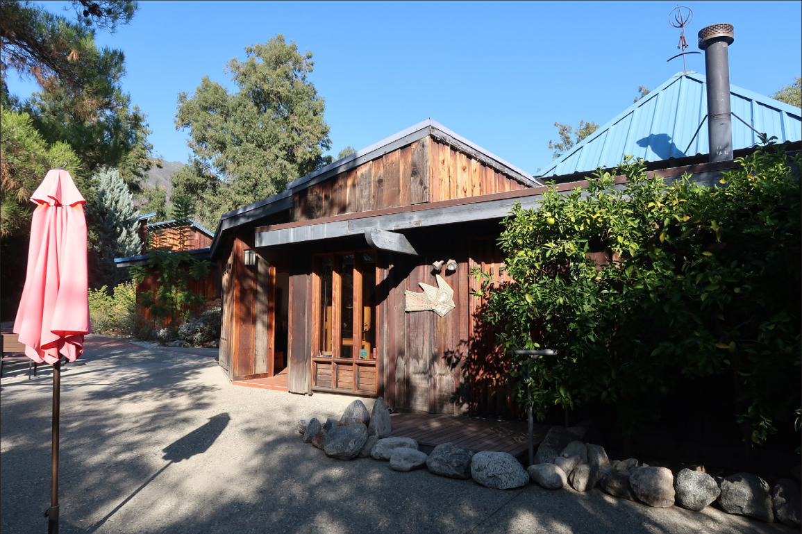
Image 2: Main House, view northeast (Chattel, 2022)
