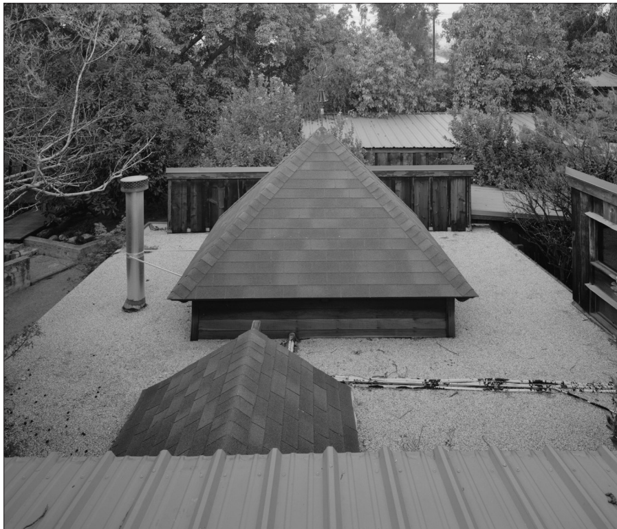
Image 16: Main House, roof, view south (HABS, 2003)
