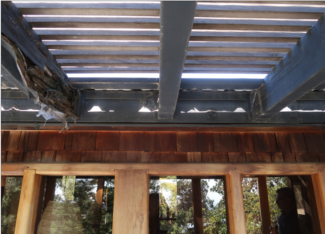
Image 17: Detail of rafters at south balcony, view north (Chattel, 2022)
