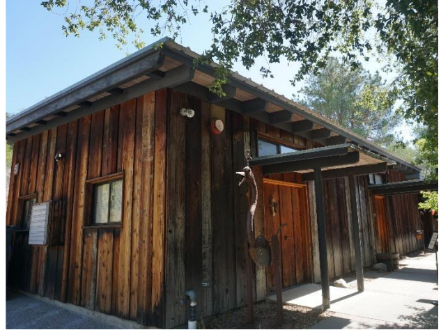
Figure 13. Current view of Workshop 2 metal roof perimeter from walkway level
