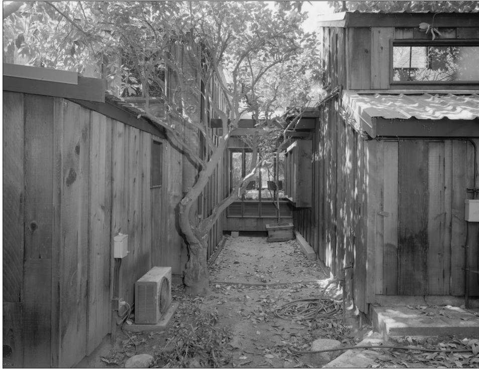
Image 5: Main House, east elevation, view west (HABS, 2003)
