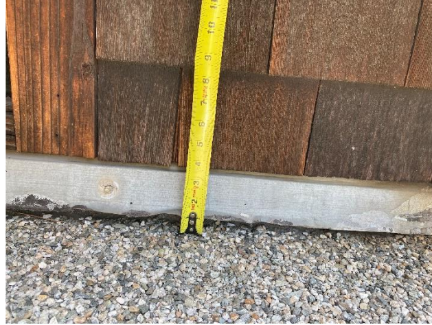
Figure 11. Shingle siding with minimal clearance at the Main House (east)
