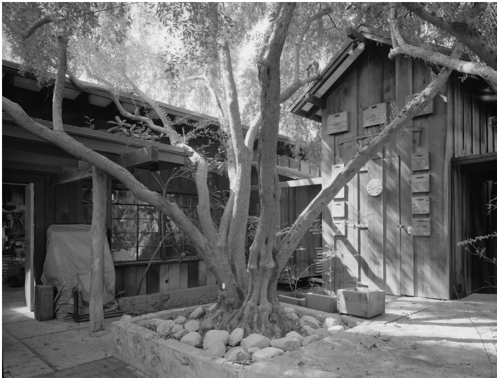
Image 2: Workshop 1 north elevation (left) and west elevation (right), view west (HABS, 2003)
