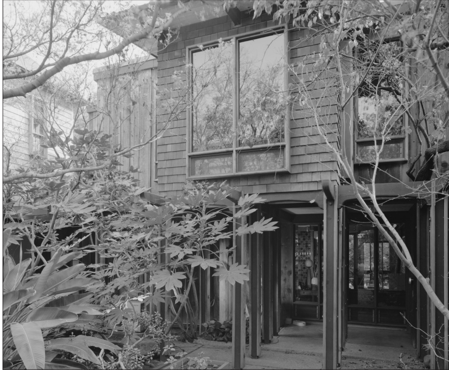
Image 13: Main House, north elevation, view south (HABS, 2003)
