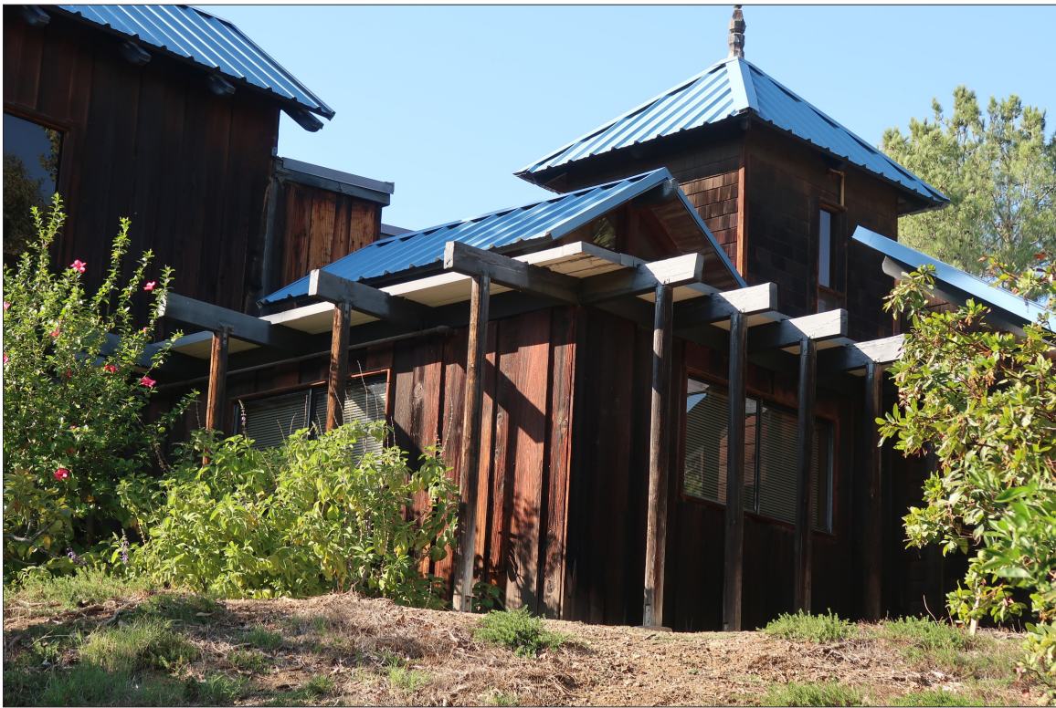
Image 12: Main House, south elevation (left) east elevation (right), view northwest (Chattel, 2022)
