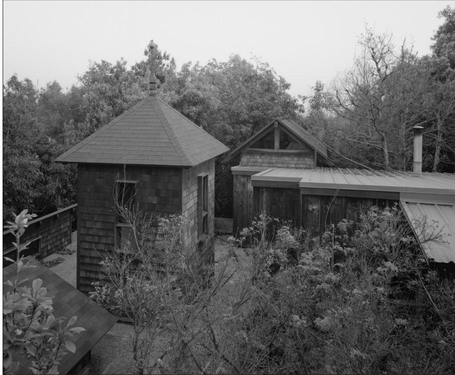
Image 15: Main House, roof, view southeast (HABS, 2003)
