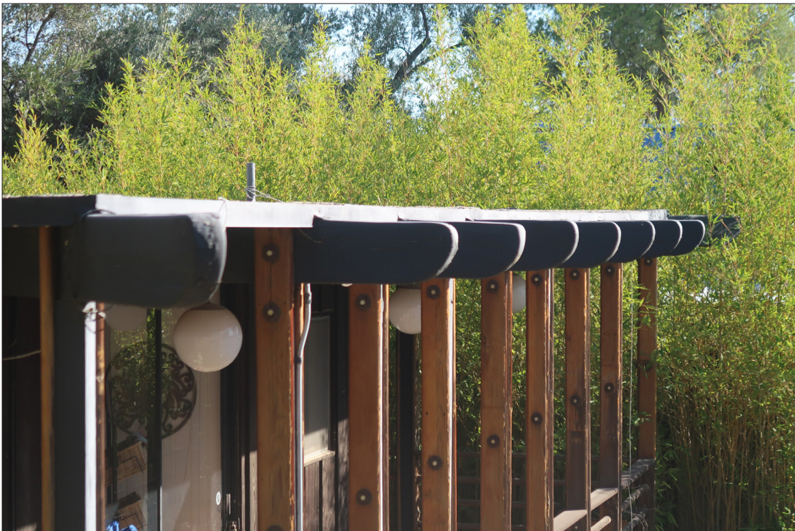
Image 30: Detail of rafters at Guest House roof (Chattel, 2022)
