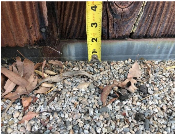
Figure 8. Vertical siding with minimal clearance at the Workshop 1 West Addition
