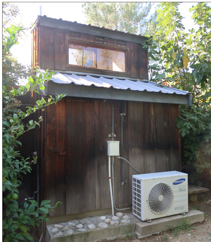
Image 14: Main House, east elevation, view northwest (Chattel, 2022)
