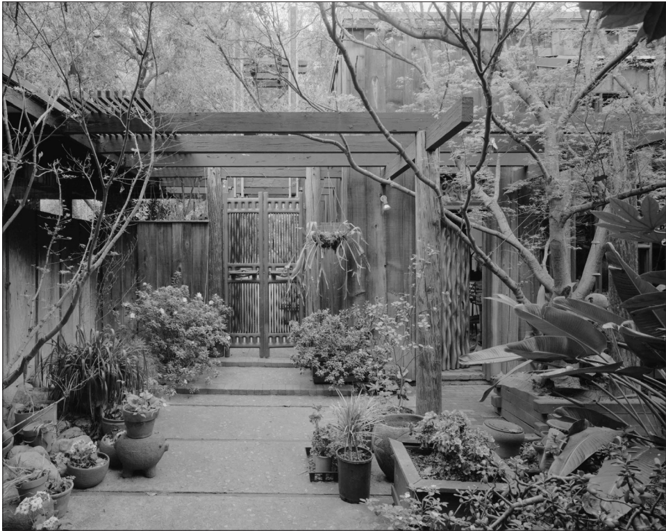
Image 12: Main House, inner courtyard, view north (HABS, 2003)
