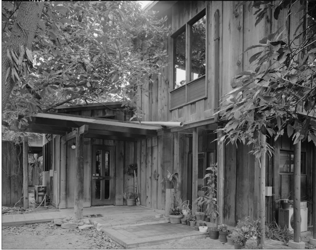
Image 9: Main House, south elevation (left) and north elevation (right), view north (HABS, 2003)
