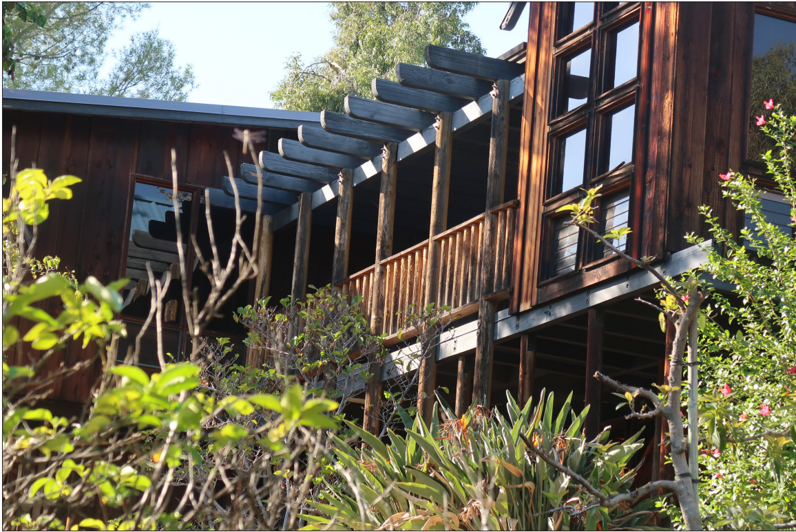
Image 11: View of second-floor south balcony, view northwest (Chattel, 2022)
