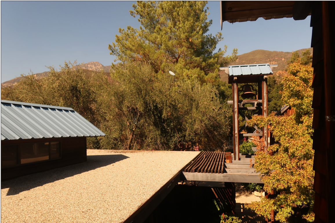
Image 21: Main House, built-up asphalt roof with gravel surfacing, view north (Chattel, 2022)
