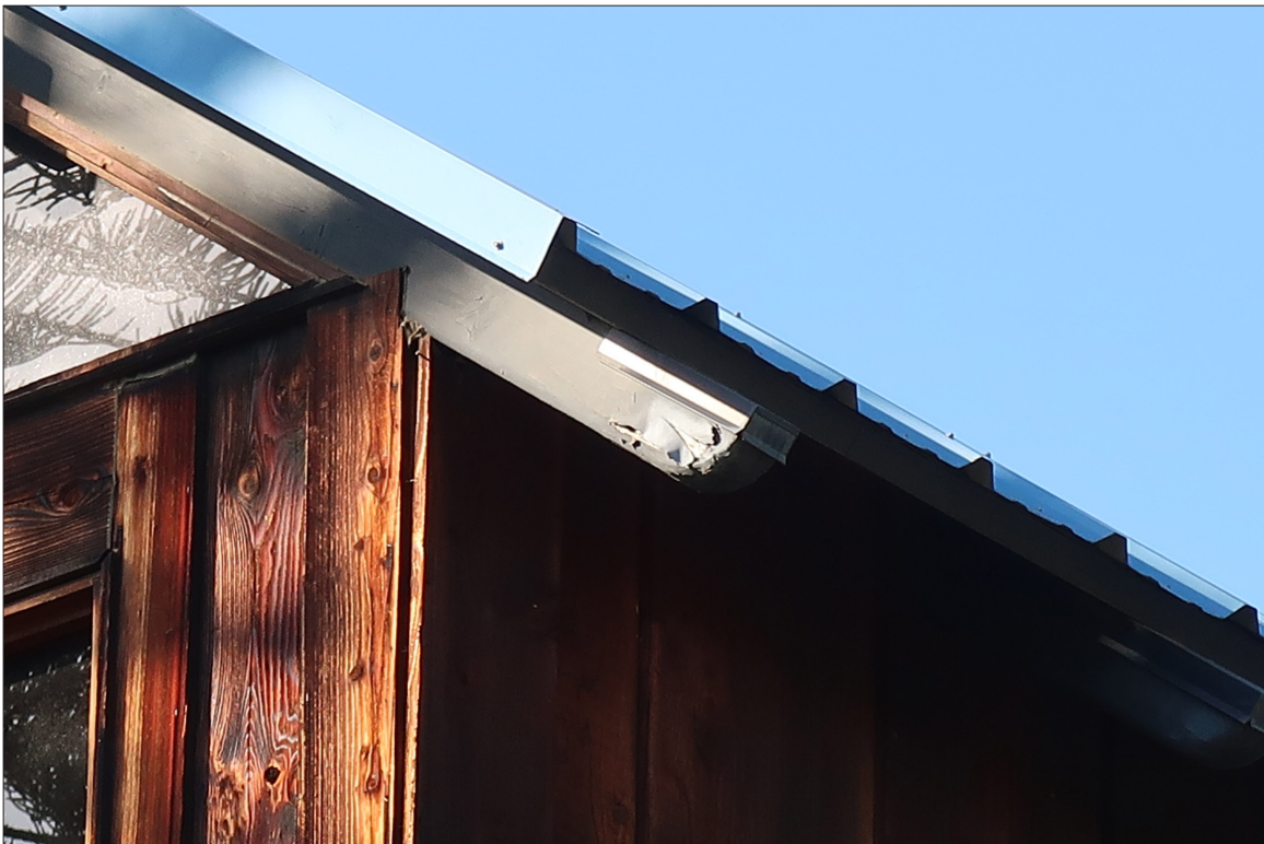
Image 10: Detail of metal cap on rafter tail, view northwest (Chattel, 2022)
