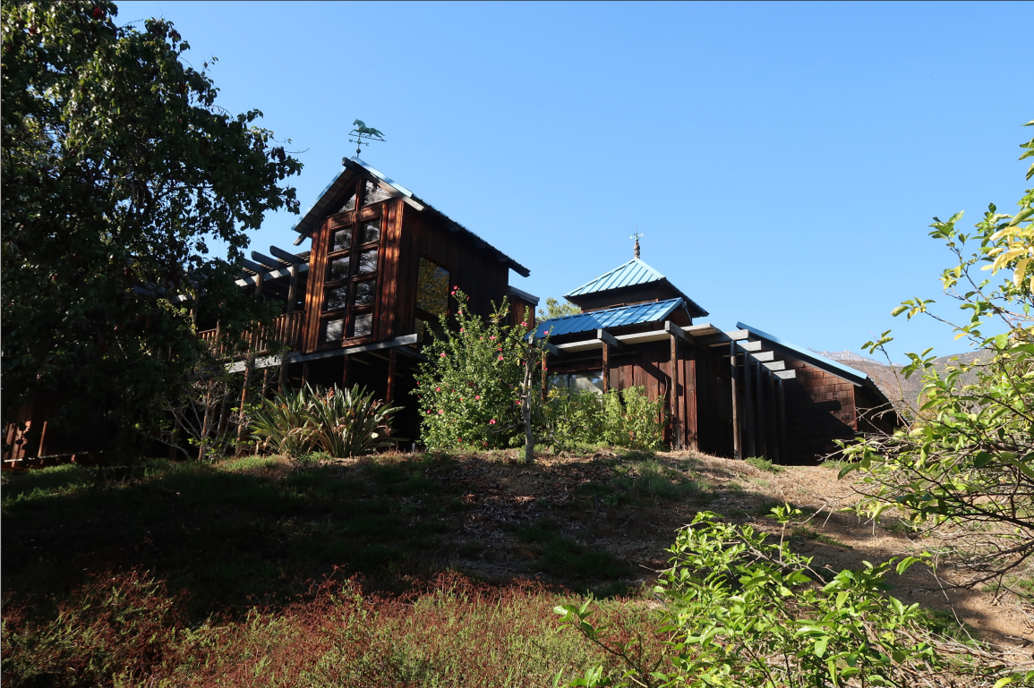
Image 8: Main House, south elevation, view northwest (Chattel, 2022)
